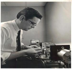
Figure 2 Stickley inserting ruby rod with silvered flat ends into laser head
