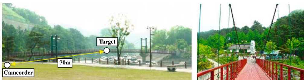
Fig. 16 A pedestrian suspension bridge. 75
