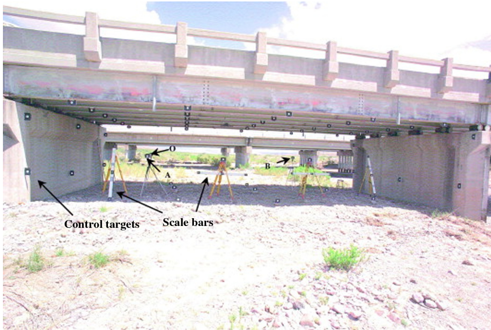
Fig. 11 Quasistatic deflection measurement based on close-range photogrammetry. 48
